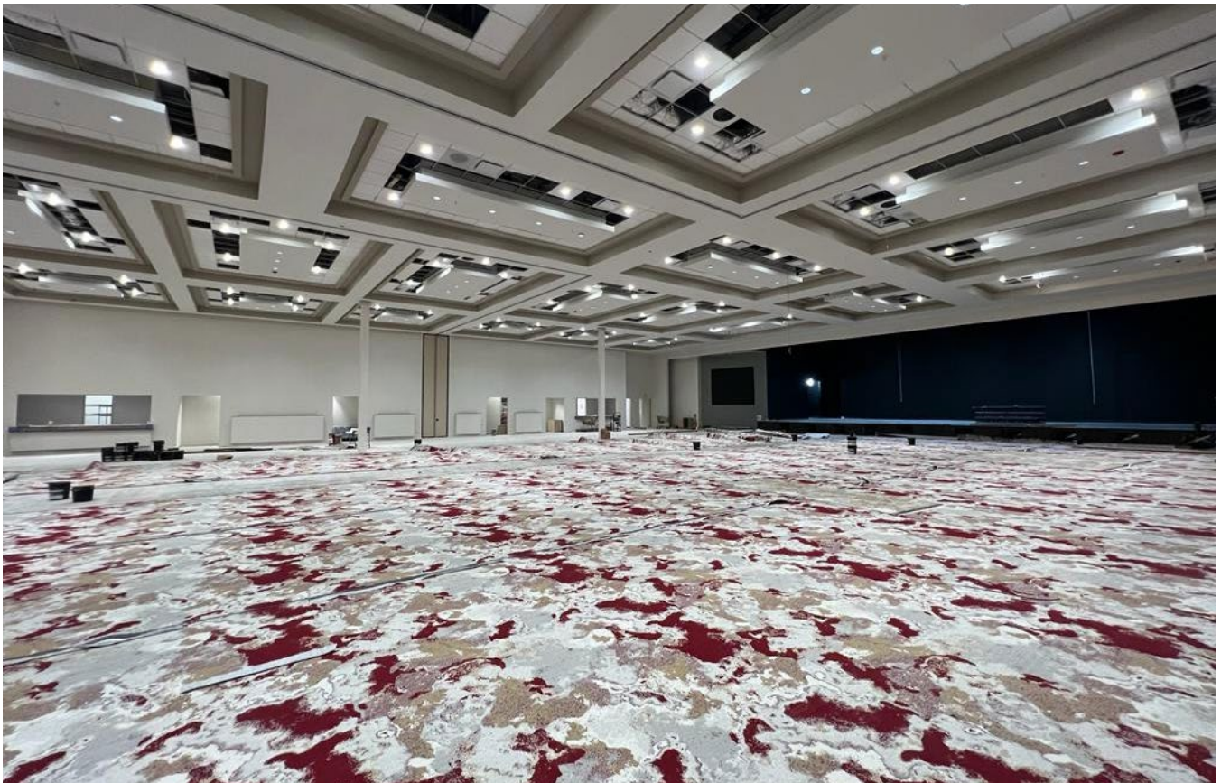
The Matrix Club Under Construction
