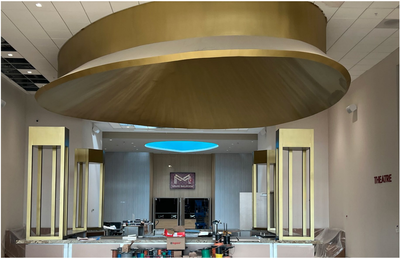
The Matrix Club Under Construction
